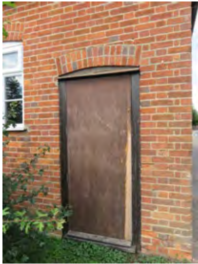
Village Hall rear door
