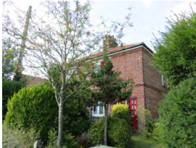
Semi-detached local authority house on Holt Road
