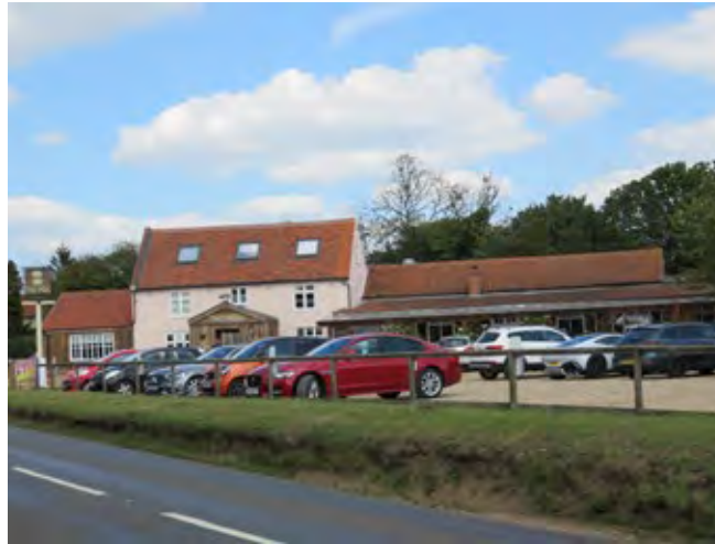
The Pigs public house, previously The Frere Arms. The pink building is the historic core whilst the rooflights are recent additions
