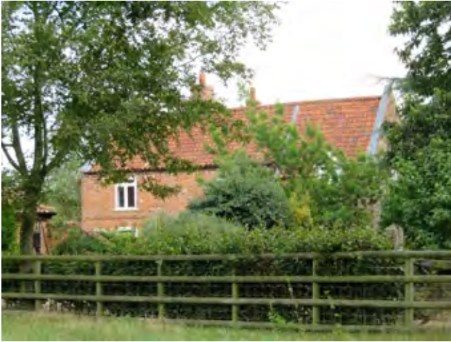
Church Farmhouse glimpsed from Sweetbriar Lane
