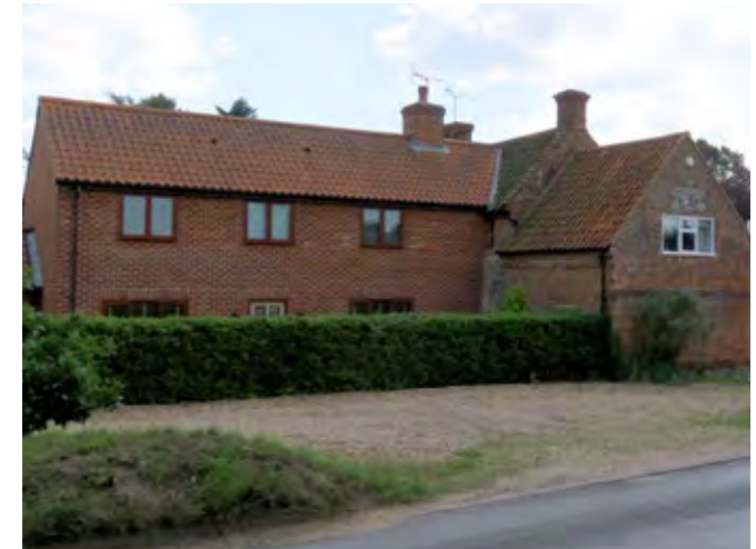
Modern extension on Green Farmhouse located north-west of Norwich Road
