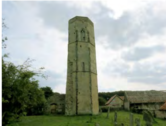
Old Church tower
