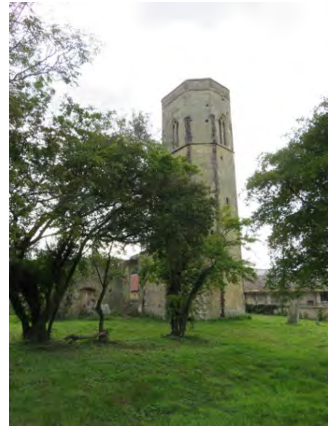
The former Church of St Peter and St Paul
