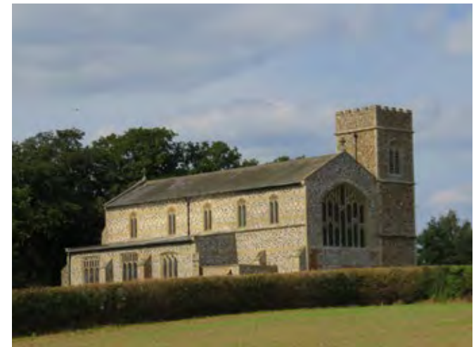
South and east elevations
