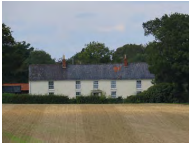
Front elevation of Manor Farmhouse
