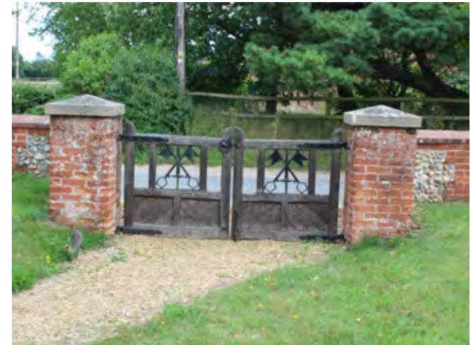
Timber and iron decorative gate to the churchyard
