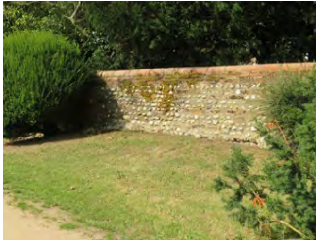
Historic flint wall with brick capping
