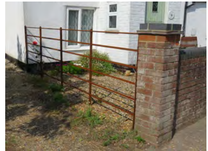
Historic metal railings
