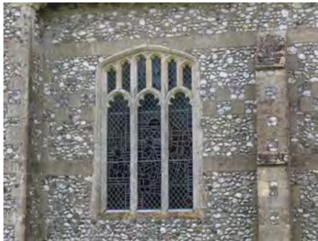
Perpendicular tracery window with stained glass
